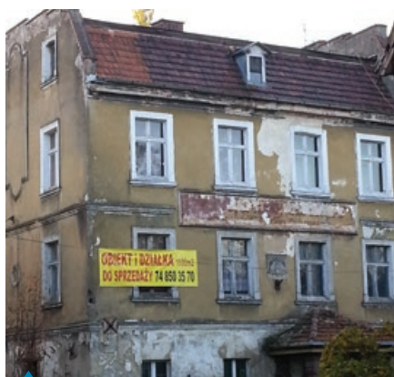
Old, pre-war building in Krzyżowa.
