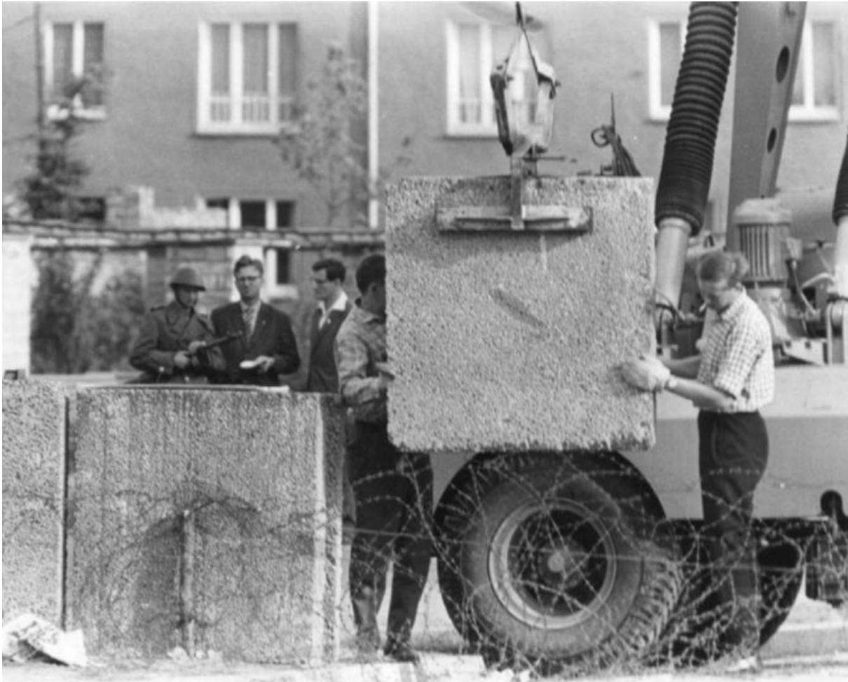
Construction of the Berlin wall with concrete blocks. August 1961.
